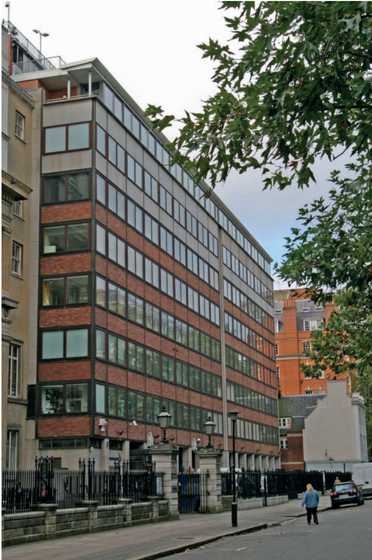
Figure 3. The Imperial Cancer Research Fund Laboratories (Cancer Research UK from 2002), 44-46 Lincoln's Inn Fields abutting RCS England, completed in 1963 , photograph 2008. It was acquired by the London School of Economics in 2013 and demolished in 2018.
