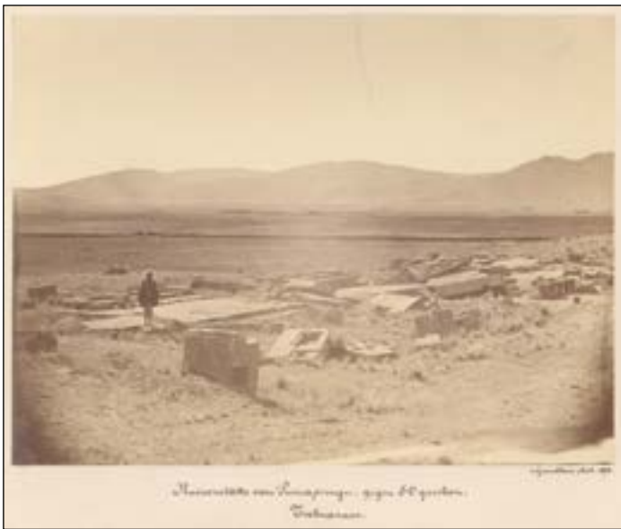
Fig. 13.6 “The Ruins of Pumapungu”, view to the southwest. © Stübel’s Collections, Leibniz-Institut für Länderkunde, Leipzig, all rights reserved.
